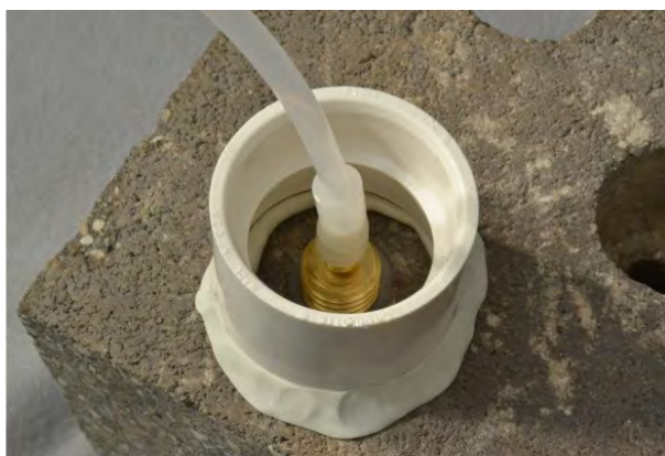
Figure 6. Water dam used for leak detection.
